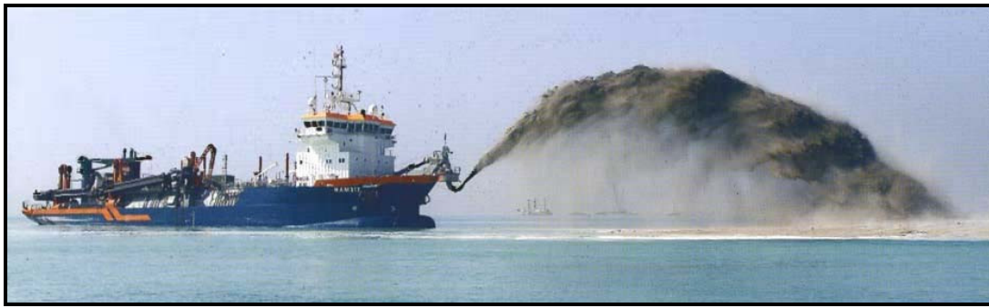
Figure 11. Trailing suction hopper dredger pumping at least 50 m from the bow
