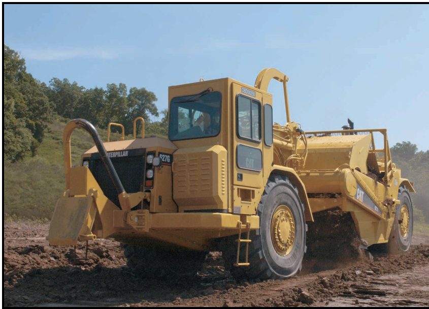
Figure 8. Wheel Tractor Scraper spreading material (Caterpillar, 2011)
